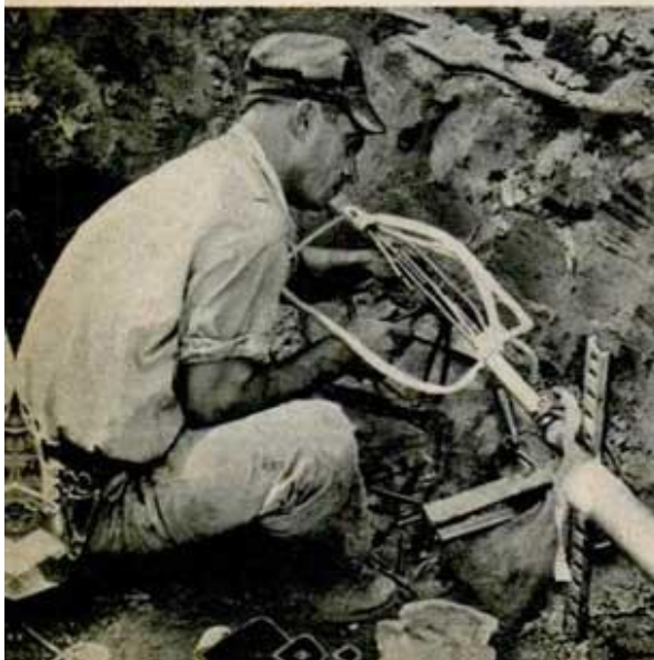
Splicing a coaxial cable, below left. At right, new cable carries six coaxials, many ordinary wire pairs
