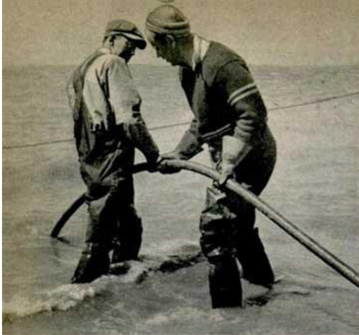
Workmen grapple with one end of telephone cable laid under water
