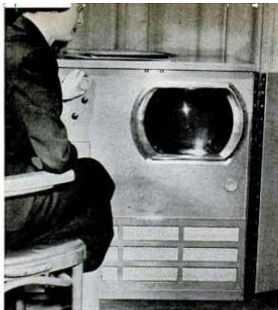
When sets with the color built into them become available—probably in six months or so—they may look like these experimental models designed by CBS engineers. The color disk is completely enclosed, folding aside when the receiver is switched to black-and-white telecasts.
