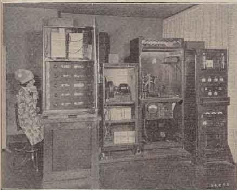
Side view of sending apparatus with cabinet doors removed. With the exception of the photoelectric cabinet at the left, the apparatus is identical with that used for monochromatic television.
