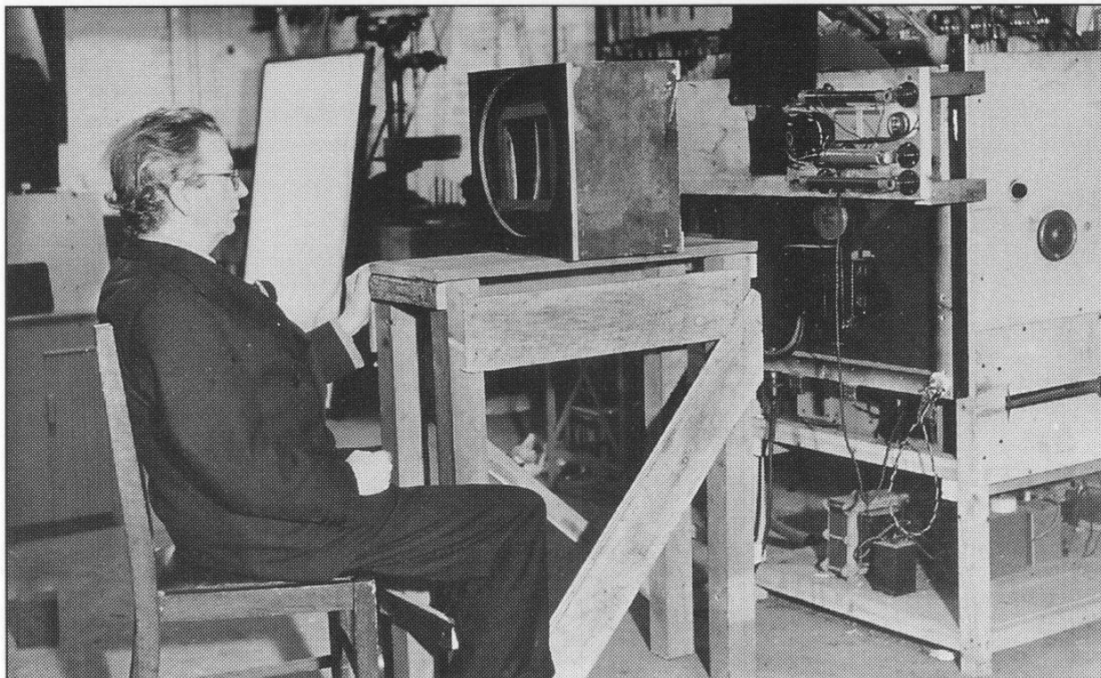
This equipment provided stereoscopic television pictures in colour. The image forming lens is in the box in front of J.L. Baird.
