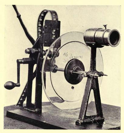
The prismatic ring can be rotated to follow any moving object; e.g., a motion picture film; or if fitted with a high-reading automobile speedometer the speed of an airplane or dirigible can be read directly off a dial by the navigating officer.
