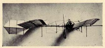
The Langley tandem monoplane with cambered wings
