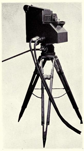
Fig. 24. The Iconoscope Pick-Up Camera Complete
