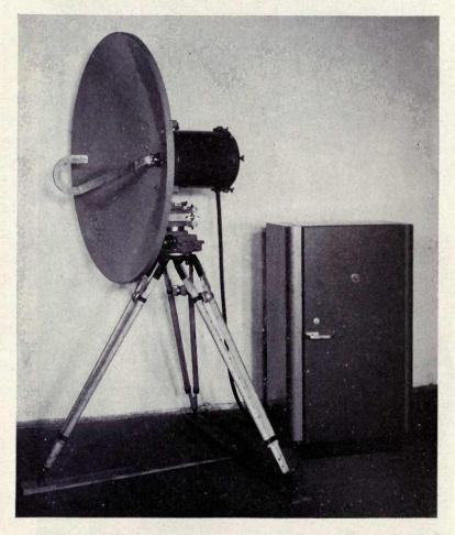
Micro-wave receiver, located in the black hub behind the parabola, used in relay links.
