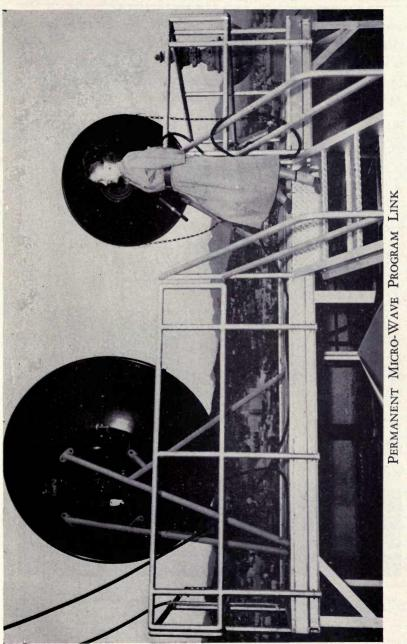
These parabolic reflectors are constantly pointed toward Mt. Wilson from KTTV-CBS, Hollywood, to carry program to the transmitter. Cables are flexible co-ax from studio control downstairs.
