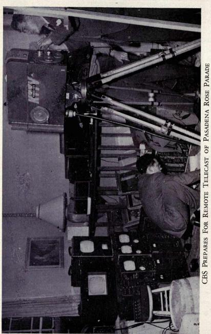
Last minute check of cameras and equipment before famous New Years Day event. Viewing equipment set-up is in house along the way. Truck, parked outside, transmits picture to Mt. Wilson via micro-wave link.
