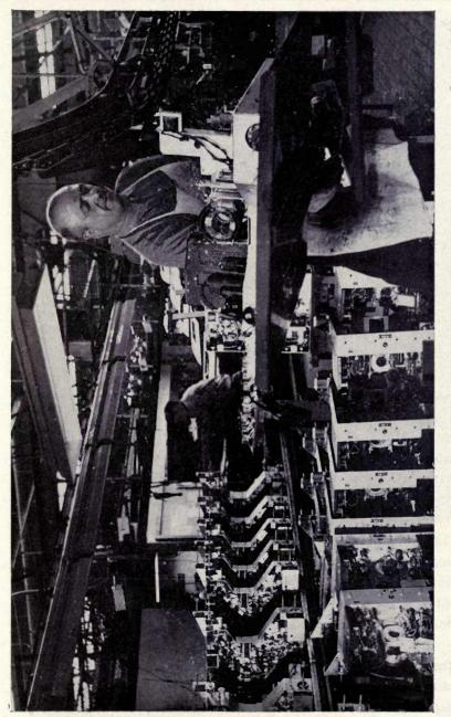
Conveyor belt brings completed chassis to workman who unloads them for final inspection and placement into cabinets.
