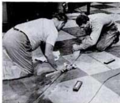
STUDIO TROUBLES arise as floor buckles under the hot TV lights. Heat also plagued commercials, melting the icing on a layer cake and making cherries run out of cherry pie.
