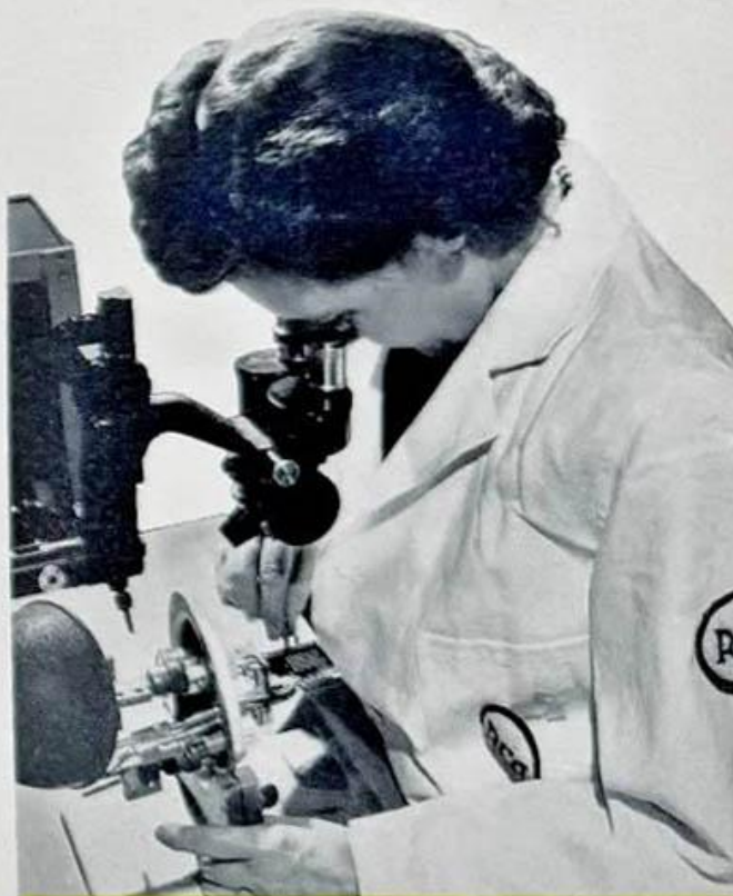
So precise is the design of the RCA 5-kilowatt television transmitter tube that the finely separated parts must be aligned under a microscope.
