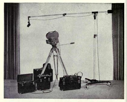
Fig. 3-4. Group of Auricon camera and sound equipment.
