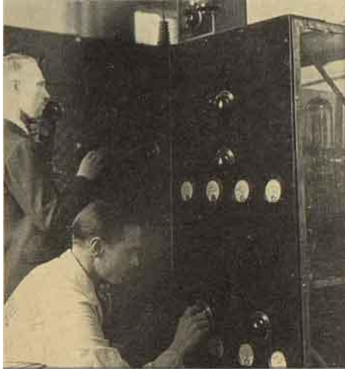
TRANSMITTER OF W9XAL—Designed and constructed by the engineering staff of First National. Student engineers are given instruction in the construction, operation and maintenance of television transmitters. This one is crystal controlled and designed for television.
