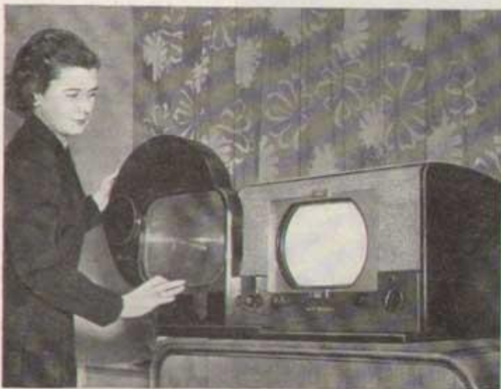
If you own a black-and-white set and CBS color is authorized by FCC, all you will need to pick up pictures in full color is an adapter like the one this girl is sliding in front of the set. Circular case contains a color wheel. Cost of unit: About $75
