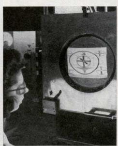
The final step is testing. A special pattern made up of Indian heads, lines, numbers, and letters was designed by engineers to indicate a tube's ability to produce a clear image. If this inspector is satisfied with its performance, it is ready to be assembled into a television receiver—and to bring you the prize fights.
