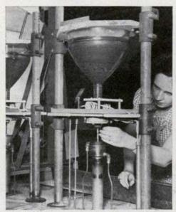
Terminals are connected to a power line before tube enters the exhaust machine, so that the elements can be turned on, insuring good vacuum. During the 64-minute trip through this device, pressure inside the tube is reduced by steady pumping to 10,000 million times less than outside pressure.
