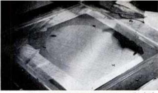
3 REMOVED FROM PHOTO PLATE, stencil is laid on wire supporting screen in frame. Shadwar mask itself cannot be used as stencil because phosphors must be spaced for "angle shots" from electron guns. Photo process assures such spacing.
