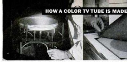
1 PHOSPHORING the face of a developmental color TV tube for a home receiver starts in darkroom. Design of shadow mask—through which electron guns shoot at colored phosphors to produce picture—is photographed on sensitized glass.
