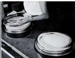
PARTS GO TOGETHER on flanged tube body. Shadow mask is first. Then come phosphored plate, a mask for outside of tube face and a glass face plate. Inside of tube body has been painted with graphite.
