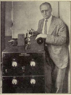
(Courtesy of the Westinghouse Electric and Manufacturing Co.) FIG. 70 a.—Westinghouse facsimile transmitter.
