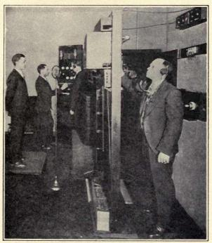
(Courtesy of the Bell Telephone Laboratories, Inc.) FIG. 98.—Television transmitting apparatus in the studio at Whippany.
