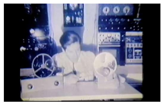
Two color wheels. The one on the left is placed in front of the camera, the one on the right is in a receiver
