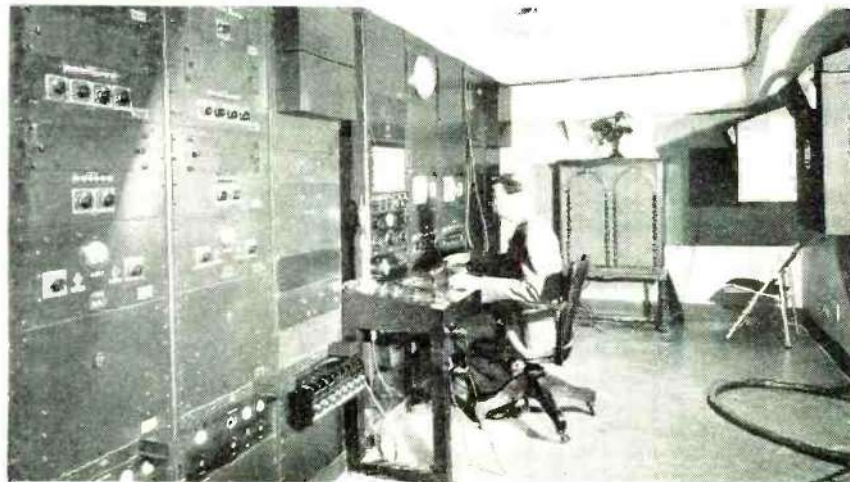
NBC Empire State Bldg. Studio television control room. A lot of equipment, but only intermittent programs. When will this equipment get regular use?
