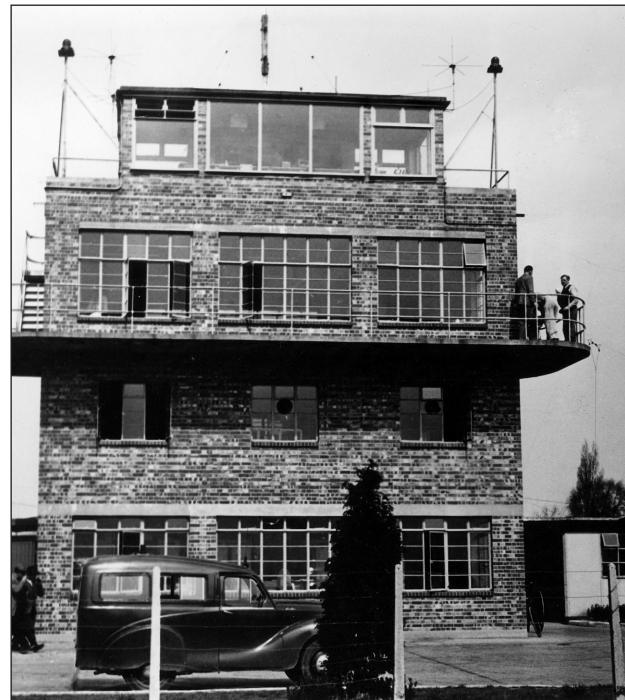
Figure 3. The old control tower at London's Heathrow Airport. Our operating space was behind the second floor windows.
