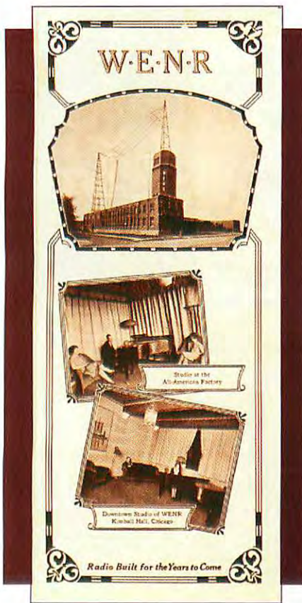
■ This 1925 photo shows the WENR transmitter towers on the roof of the All American Radio Company's manufacturing facility.
