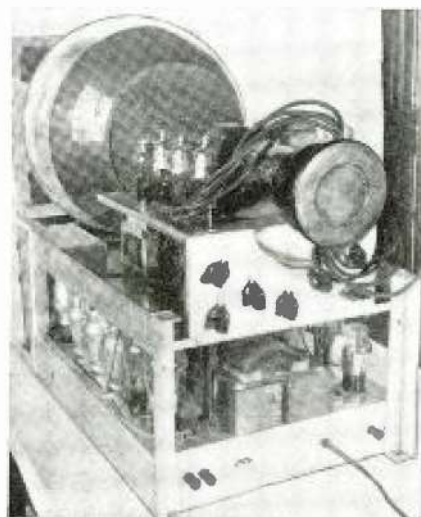
Two chassis views of the DuMont Set. Double decks are used for compactness.
