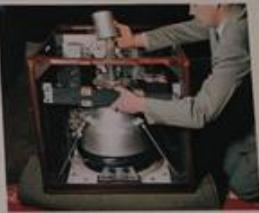
Figure 4-9 — Installing the Yoke and Neck Shield Assembly
