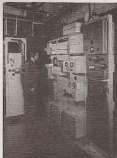
The apparatus which raises the video frequencies to a suitable value for transmission.
