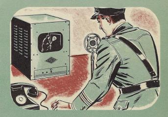
The ''Utiliscope'' camera is sensitive to infrared light which is invisible to the human eye. Safes, show cases, etc., when illuminated by infrared at night, are apparently in total darkness, yet every detail is visible on the ''Utiliscope'' viewing screen. A watchman placed in another room can observe a number of scenes. Any intruder shows up at once. Security possibilities for banks, stores, museums, etc., are tremendous.
