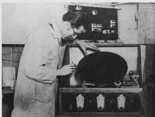
Fig. 46. Pilot scanning disc television under construction. (Edgar H. Felix, Television, Its Methods and Uses , p. 144)
