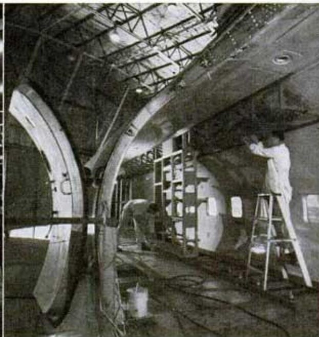
RACKS for five tons of electronic gear are installed in a converted DC-6, one of two which will be used in Stratovision flights.
