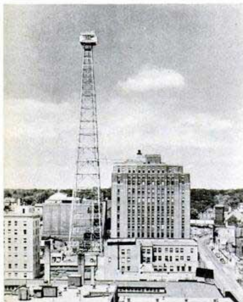
TALLEST TOWER in the cross-country microwave-relay system that will carry TV convention programs to the audience west of Chicago is this lofty structure in Des Moines.
