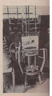
Here is one of the most difficulty problems in the early stages of metal tube production: sealing glass face plate to metal cone. The machine is completely make matic, heats the glass to 2000.
