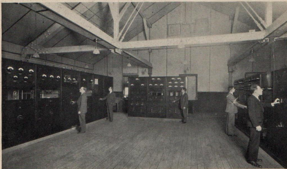
In the power room of 3XN, the Laboratories' experimental radio station at Whippany, New Jersey. On the left, a fifty kilowatt set with its power panel in the rear; on the right the five kilowatt set. At their posts for experimental operation are O. A. Keefe, R. E. Poole, J. W. Smith, W. N. Mellor and J. C. Herber
