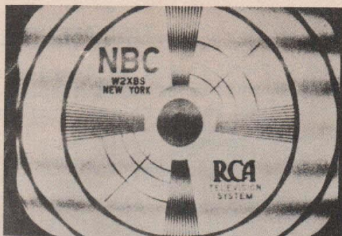
Fig. 8-Sound Modulation in Picture
